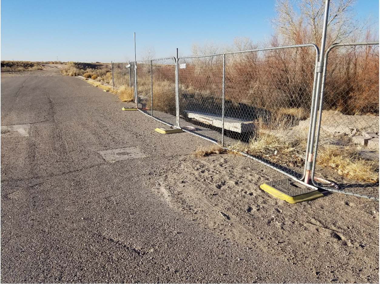
Concrete rundown: View from termination of San Lucas and Charmartin Avenues
