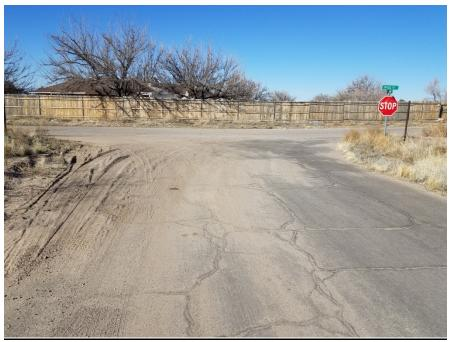
Assessment: Complete breakdown of asphalt and sub-base
