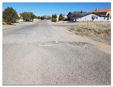
Assessment: Complete breakdown of asphalt and sub-base
