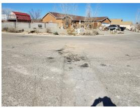
Assessment: Irregular cracking and breakdown of asphalt
