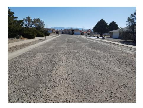
Assessment: Irregular cracking and breakdown of asphalt
