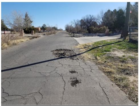
Assessment: Complete breakdown of asphalt and sub-base
