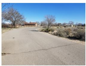
Assessment: Irregular cracking and breakdown of asphalt
