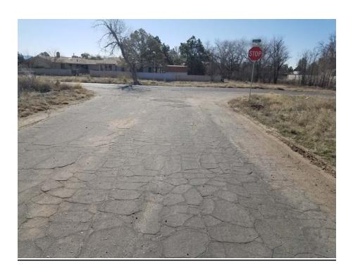
Assessment: Complete breakdown of asphalt and sub-base
