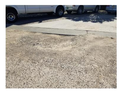
Assessment: Complete breakdown of asphalt and sub-base
