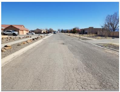
Assessment: Irregular cracking and breakdown of asphalt
