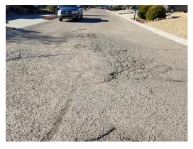
Assessment: Complete breakdown of asphalt and
