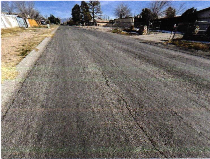
Figure 1: Longitudinal cracking
