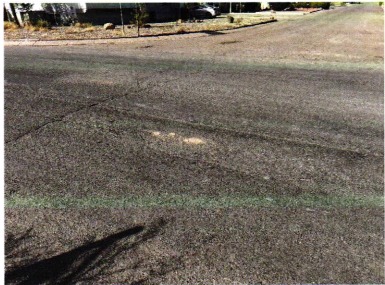
Figure 2: Transverse cracking
